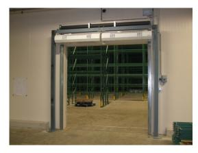
Compact AC1000/160 system for temperature and odour separation mainly used for smaller doorways.
