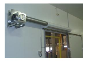
Decentralised AS355 system with possibility to connect suction side to ducting used for temperature separation.
