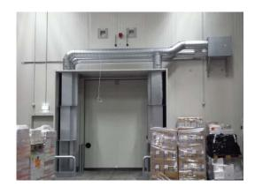
Powerstream-DS Block for maximum blocking high temperature and humidity coming into the freezer. (injection of dry air in the insulating layor can improve performance)
