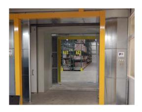
Powerstream-Airlock system. Ultimate protection with highest efficiency (only in combination with dried and conditioned front room (e.g. 2°C and < 60%RH)
