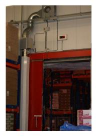
Temperature barrier at freezer door with single standing and heated decentralized AS400 for a strong airstream and minimal floor contact
