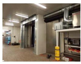
Powerstream-Comfort system. High protection in combination with minimal active dry capacity in front rooms with higher humidity level
