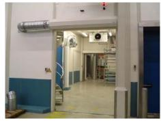
Example of airlock by use of decentralised industrial Airstop systems in combination with active dehumidification by cooling or drying
