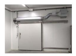
Temperature barrier at freezer door with heated decentralized AS315 – can be combined with plastic flaps
