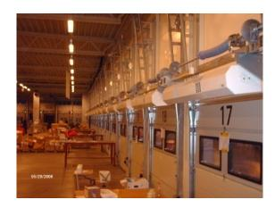
AC1000/160 system to protect outside door at conditioned area
