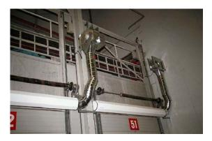
AS315 system for outside door at conditioned area
