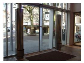
Compact 400 double standing, all components integrated in single design pillars. Stainless steel design. Form of outblow drums can be enlarged with adaption parts
