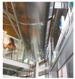
Double Ellips systems for protecting big entrances. Special attention for the cradle which fixes the outblow angle. Integrated mini bag filter.
