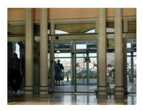
Example Airstop system for customer entrance with high resistance against wind/draught by use of double standing system.
