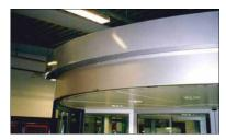
Airstop system for customer entrance adapted to revolving door shape
