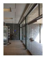
ASE400F system for customer entrance, completely integrated in technical ceiling
