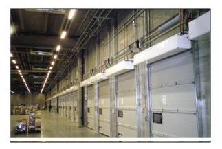
Compact AC2000 systems for protecting outside doors in combination with night heating according to dedicated zones
